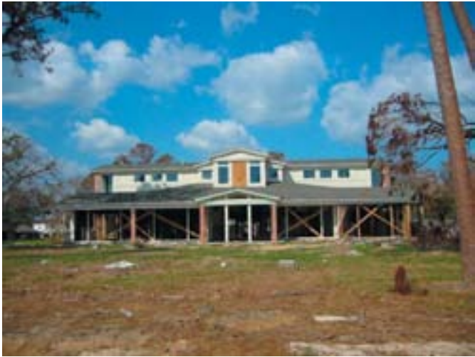
1st floor break-away walls leave upper floor intact.
