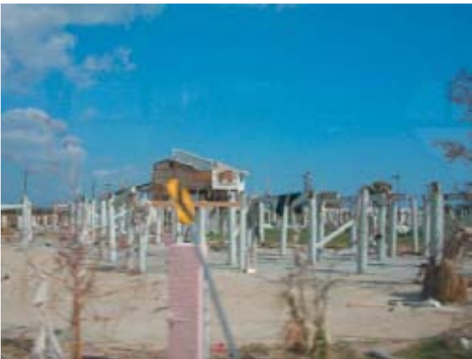
Condominium housing swept from concrete columns.
