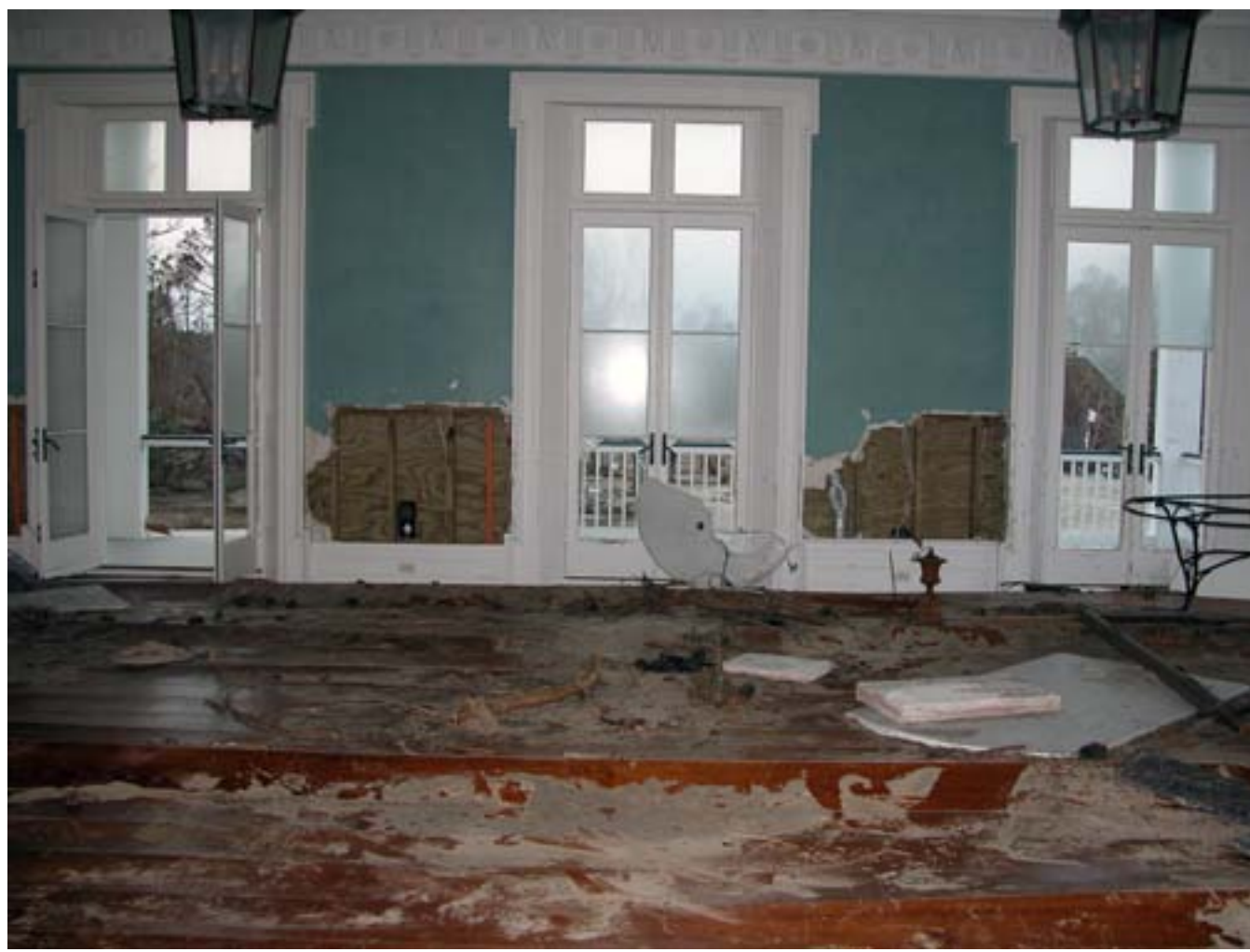
Damage in the guest house is constrained to the bottom 3' of the sheetrock and buckling of the wood flooring.
