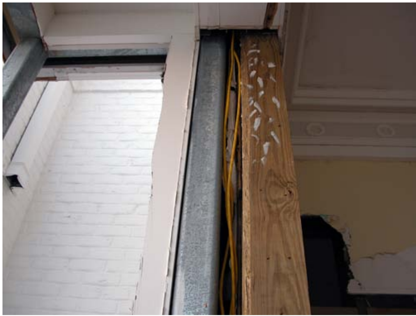
This is an interior view of steel columns embedded in the wall.
