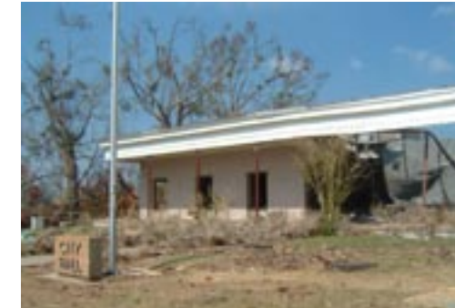
Damaged City Hall
