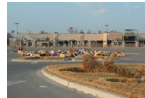
Damaged Wal-Mart store
