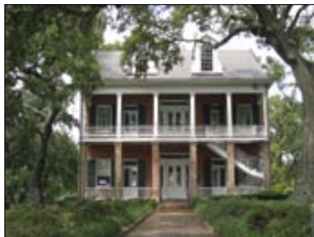
THE 1856 TULLIS TOLEDANO HOUSE IS GONE. A THREE STORY CASINO BARGE NOW SITS ON TOP OF THE SITE.
