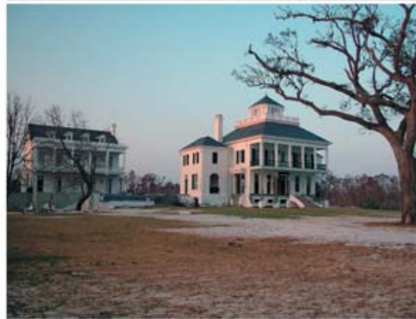
VIEW FROM JUST INSIDE FENCE
