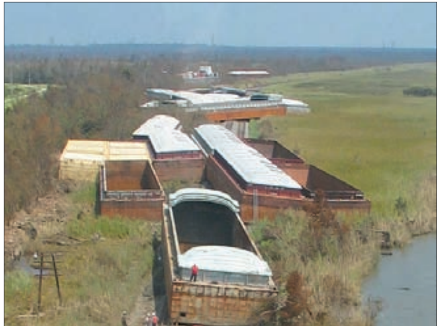
Top: Bay St. Louis bridge. Bottom: Barges washed ashore.
