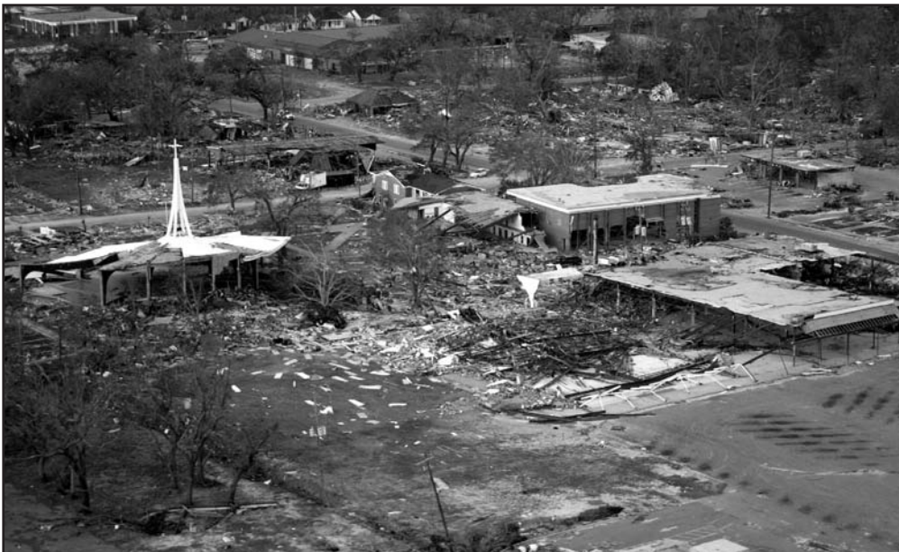
The skeletal structure of a church and other buildings in Long Beach, as photographed from a helicopter ride on Tuesday afternoon.
